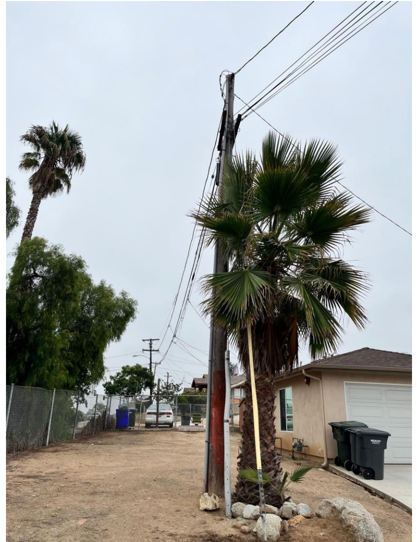
Looking south towards overhead utilities
