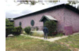
Current Accessible Entry
