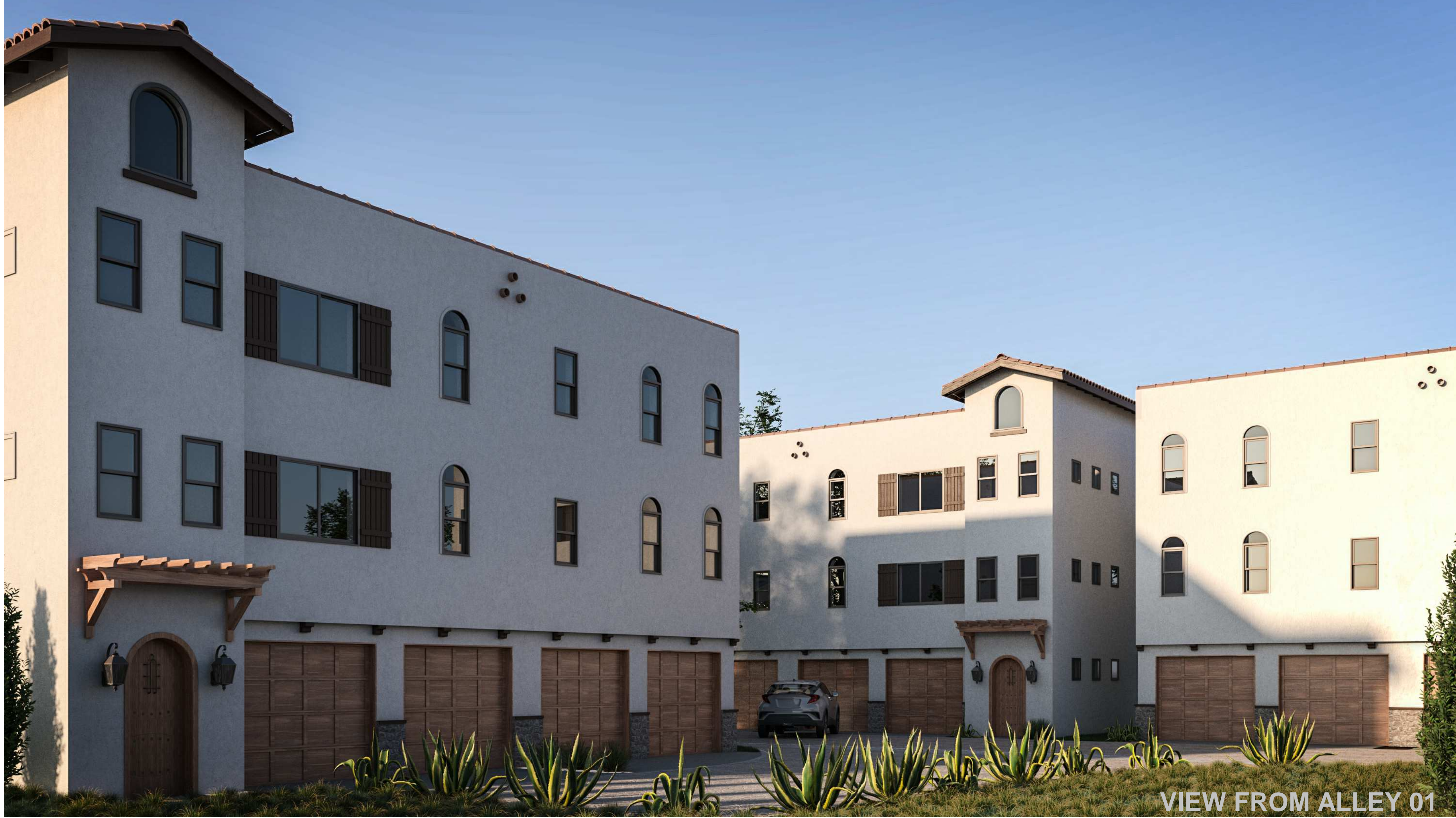
VIEW FROM GROVE STREET
