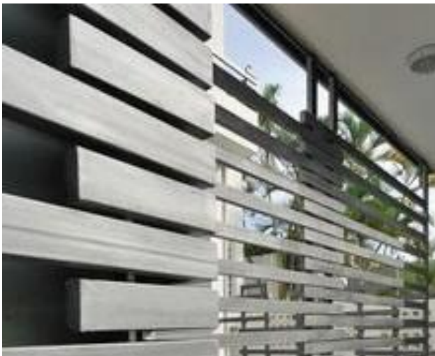
Concealing building facade treatment
