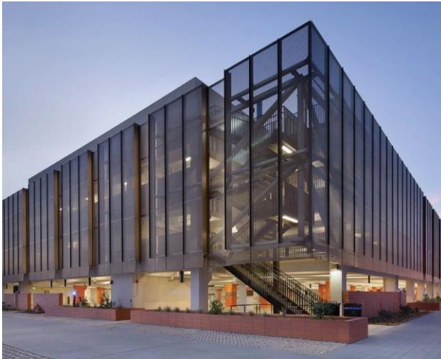
Parking structure is enhanced with an exterior screen/façade
