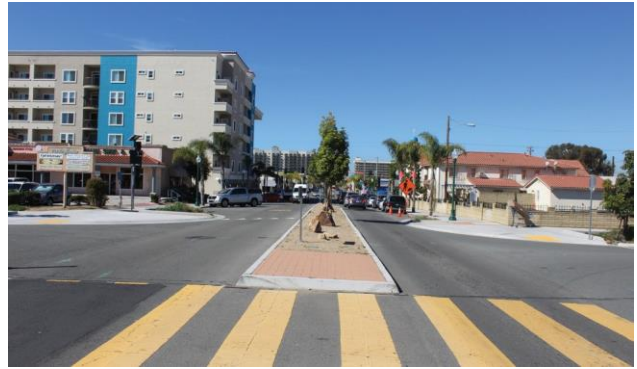
Existing main street
