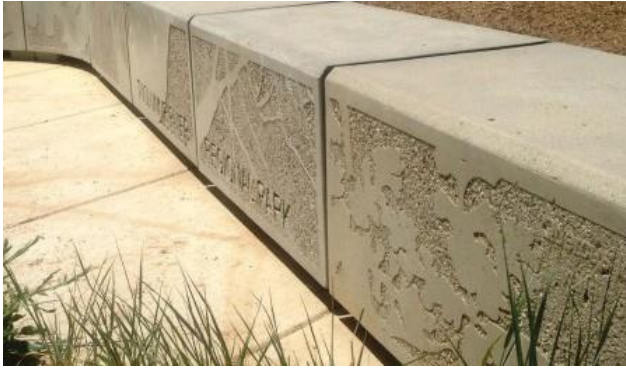
Concrete seat-wall with organic pattern
