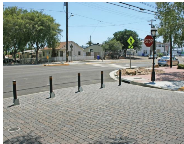
Removable bollards at the intersection of A Avenue and Plaza Boulevard
