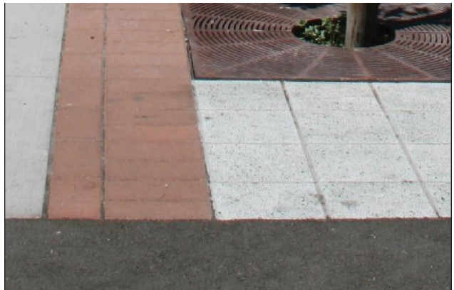
Scored concrete used with pavers and tree grate
