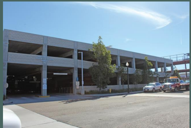
National City Education Village Parking Garage
