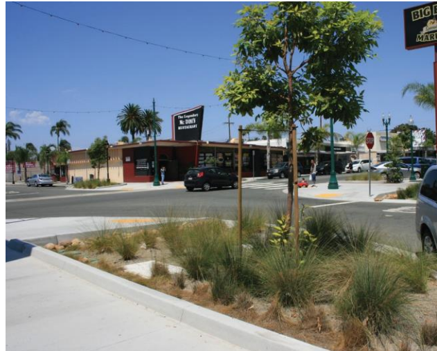
Storm-water bioretention areas along 8th Street
