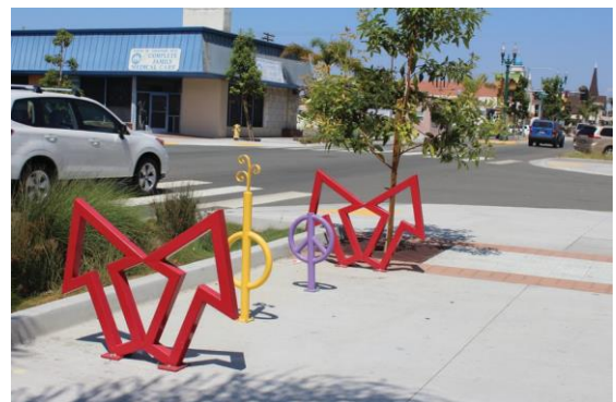
Street improvements on 8th Street
