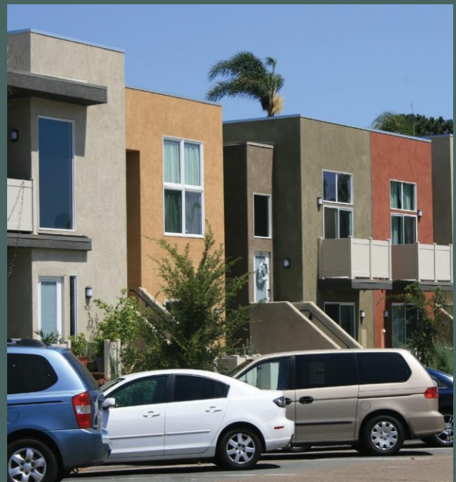
Angled Parking on C Avenue
