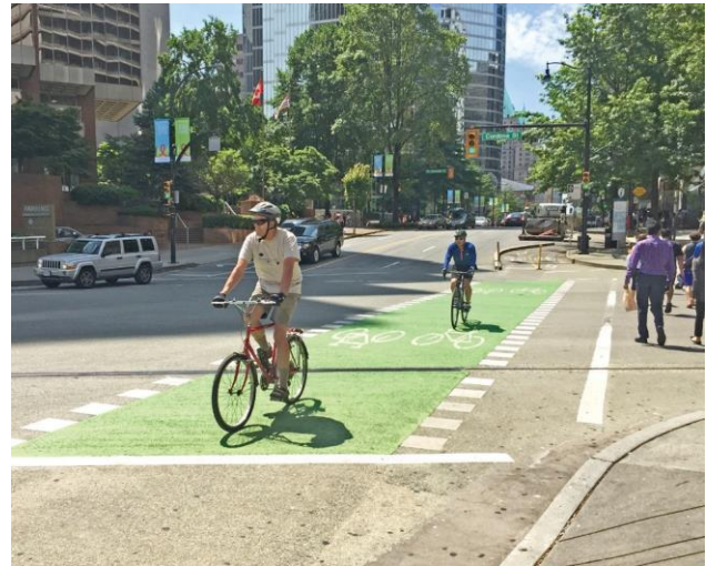
Intersection markings provide additional safety & comfort
