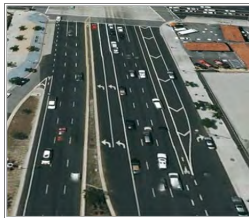
Shared bicycle-right turn lanes require warning signage as well as pavement markings.
