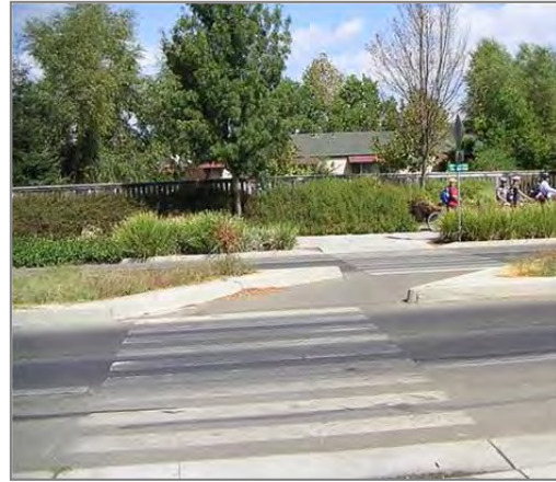
An offset crossing forces pedestrians to turn and face the traffic they are about to cross.
