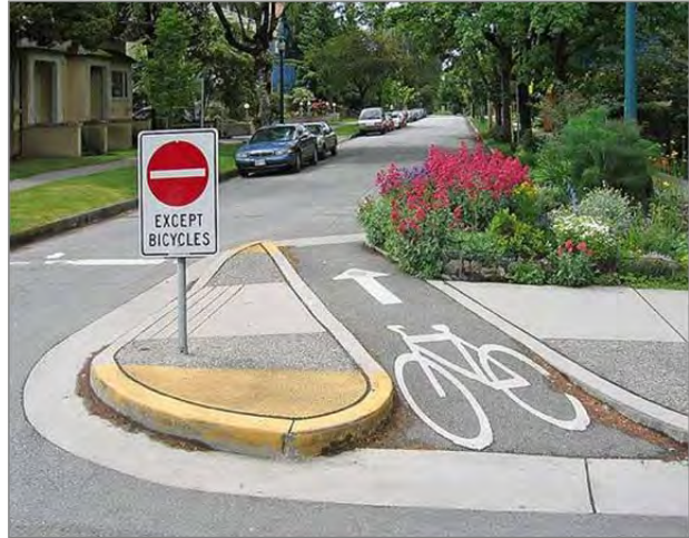
Choker entrances prevent vehicular traffic from turning from a major street onto a traffic-calmed bicycle boulevard.
