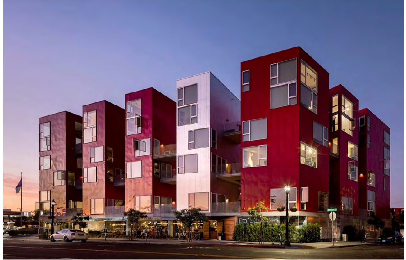
Located in the heart of San Diego's Hillcrest Village, Eitol is a mixed-use, multifamily residential building. Its 13-tower design creates unique, standalone-like units with no shared walls, and also creates the opportunity to have private and shared exterior spaces.
