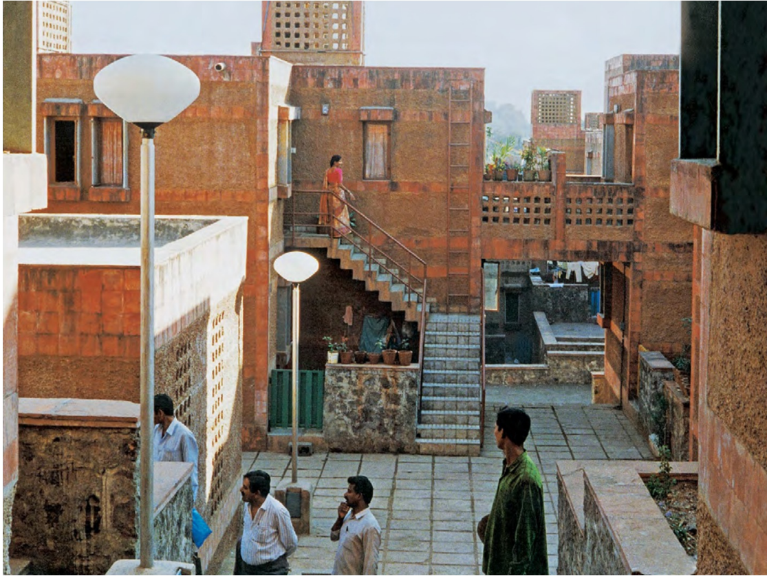
CIDCO Housing located in Navi Mumbai, has an overall density of 55 low-cost housing units per acre and was designed in a way that creates livable public space, semi-public space and private space.
