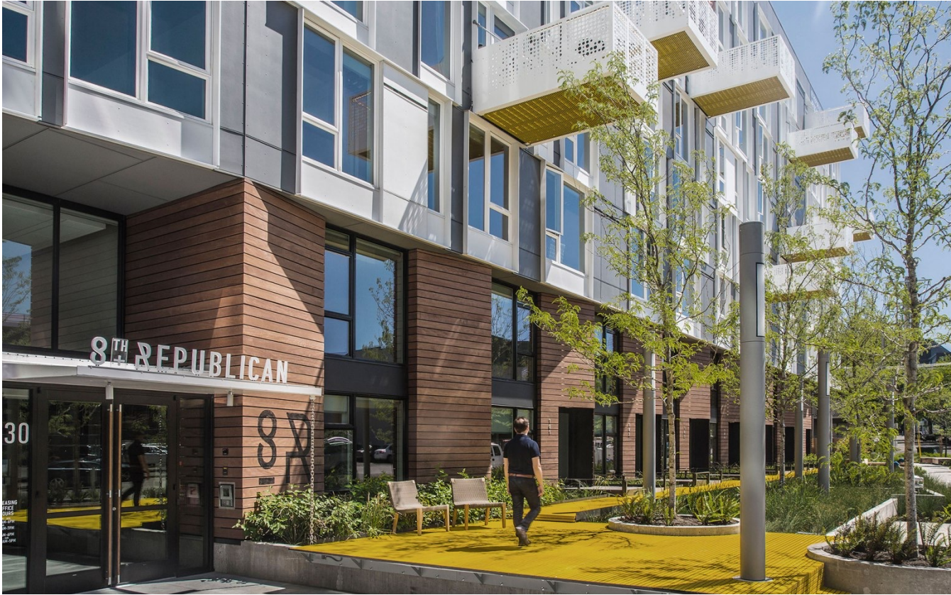
The 8th & Republican Mixed-Used Development, located in Seattle and design by Miller Hull Partnership, is set back from the street at mid-block proving a generous public courtyard, the backdrop for a well-loved neighborhood café and patio with a participatory water feature.
