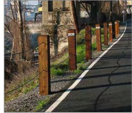
Post and wire fence.
