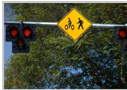
Half-signals for bicyclists should be clearly marked to minimize confusion.
