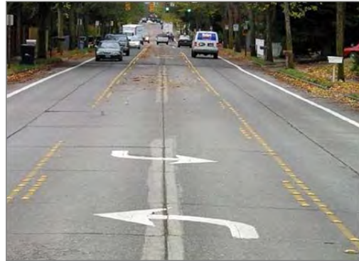
This road was re-striped to convert four vehicle travel lanes into three travel lanes with bicycle lanes.
