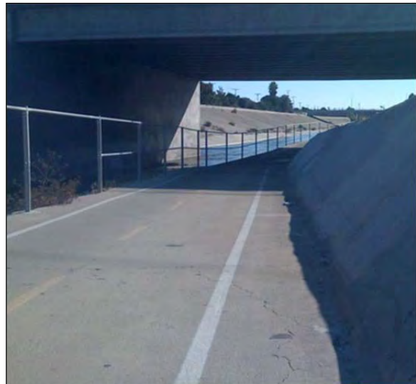
Undercrossings provide key connections and allow path users to avoid at-grade crossings of major streets or avoid barriers such as freeways and rail lines.
