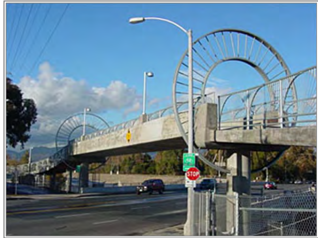
Overcrossings are frequently used over a major roadway.
