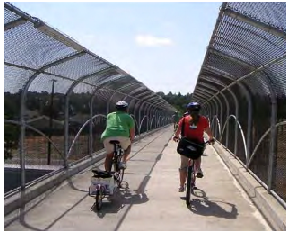
Crossing over a freeway
