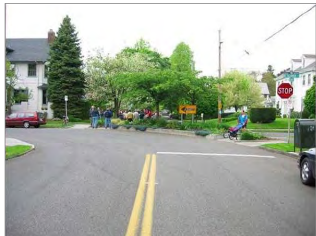
Traffic diverters prevent through-vehicle traffic as well as cross-traffic.
