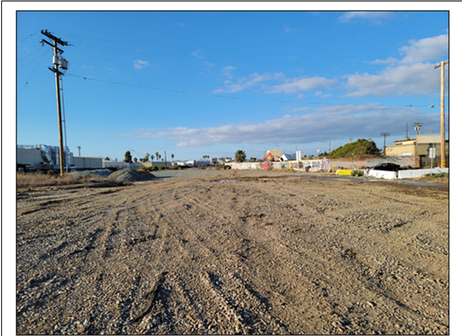
West 19th Street looking north toward location of new rail spurs (2025)
